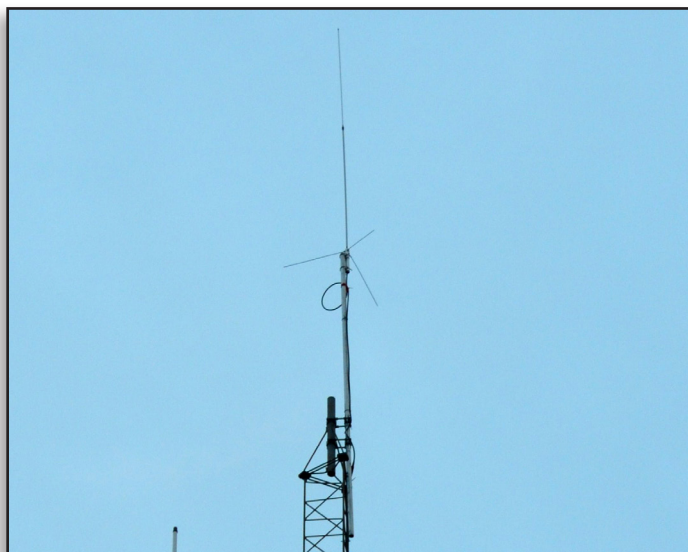
The new antenna on the top of the tower. The antenna is now roughly 90 feet above ground.
